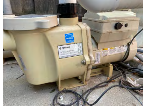
Variable Speed Pool Pump
